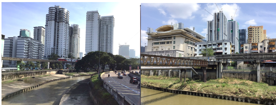
Fig. 9. Building condition along the waterfront in KL Sentral WTOD
