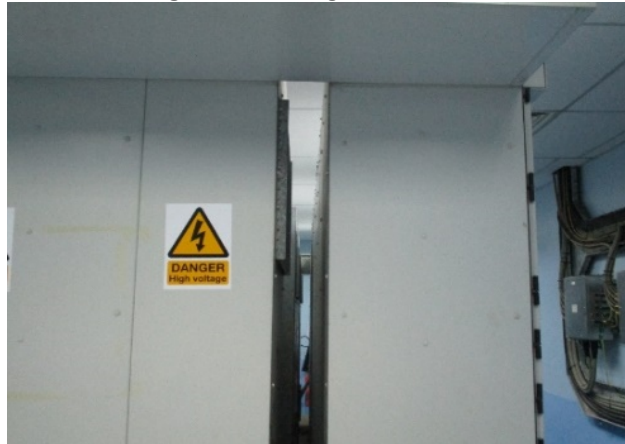
Fig. 6 Cabinets not attached/tied together which may pound on each other
