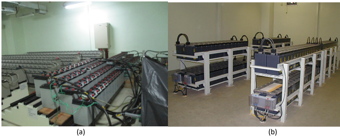
Fig. 7. (a) Batteries are not secured onto the racks (b) example of secured batteries rack
