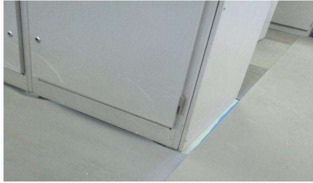
Fig. 5. Anchorage is unknown
