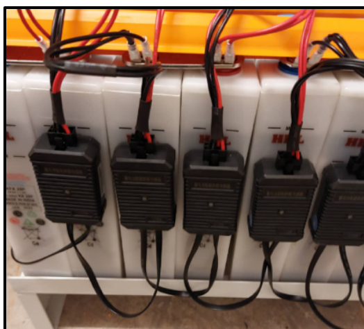
Fig. 3. Cell sensor attached to the front side of the cell
