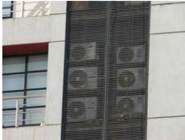
Fig. 17. Shows how the special space designed initially from the design phase enhances the overall building's aesthetics preventing AC chaotic façade
