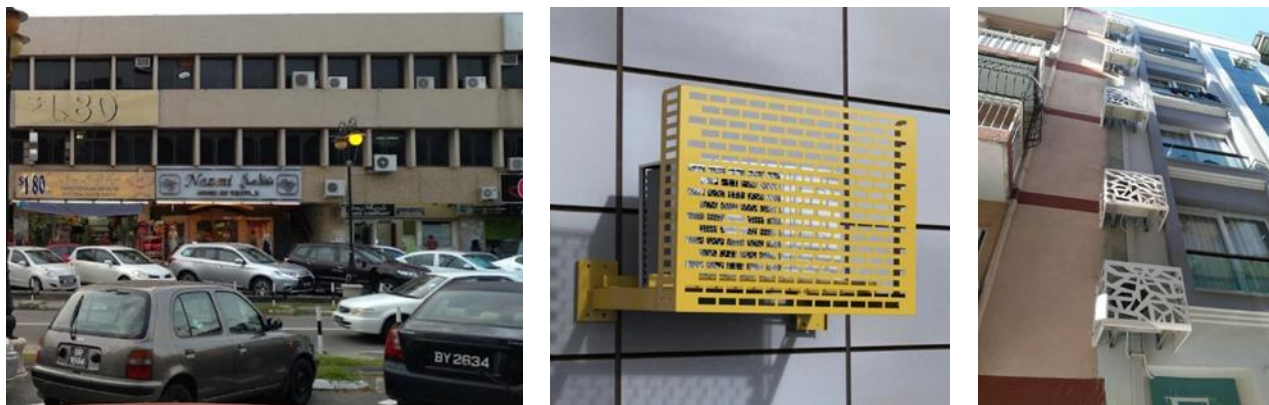
Fig. 3. Shows the exterior HVAC system model solution to inaccessible façade and how they enhance visual appeal
