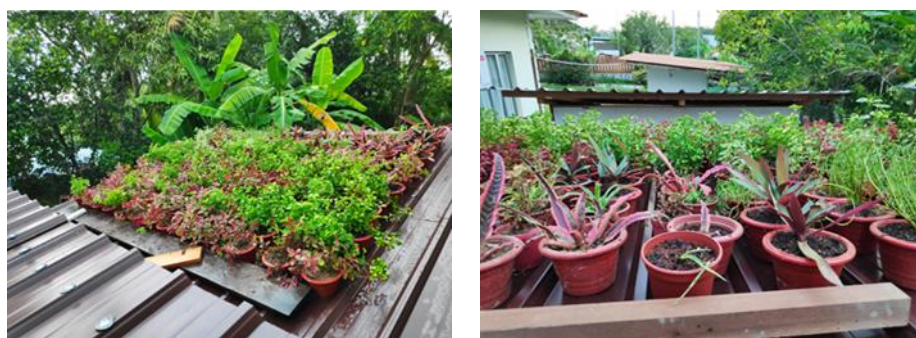
Fig. 3. Plants arrangement for the green roof setup
