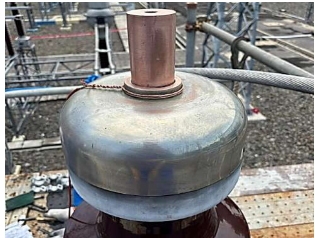
Fig. 6. The bushing conductor that has been cleaned
