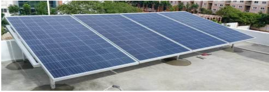
Fig. 4. Mounting 300Wp solar panels in series
